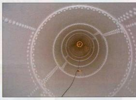
used. At the same time as the applica- View of the freshly tion, small steel plates were coated, recoated penstock on which destructive tests were sub- (originally consequently.carried out. For example, a structed in 1899). plate was cut in a transverse (vertical) An area of 1800 m<sup>2</sup> direction, and inspected using micro- was coated. (Photos scopic techniques for further investi- by courtesy of gation into the porosity of the coating General Coatings
