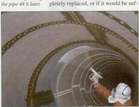
ficient to renew the corrosion treatment. Tests revealed that apart from the corrosion damage, the penstocks were in relatively good condition, and therefore it was decided to renew the anti-corrosion protection only.
