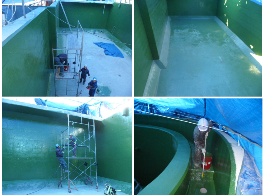
Different views on the inside of the concrete reservoir during and after application
