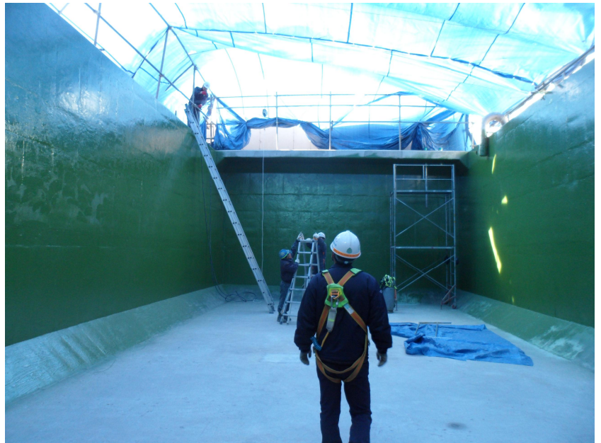
Different views on the inside of the concrete reservoir during and after application
