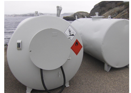
Different views on the coated reservoirs, all protected with Humidur from corrosion
