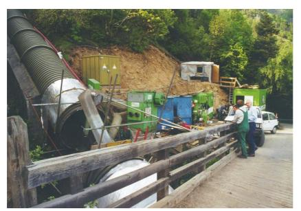
The picture on the left, which was taken after completion of both section 2 and 3, shows the installation of the site at the station in the middle without housing. In the background, you can see the winch chamber. The pulley block is fixed on the lower part of the upper pipe.
