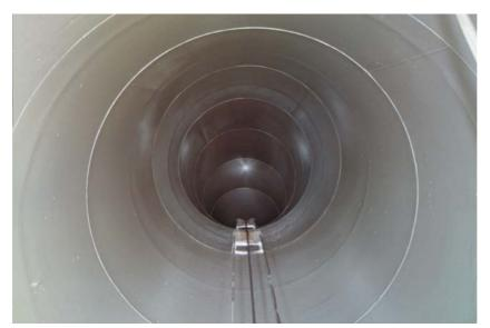
The picture on the left shows the finished first applied layer on the area of a positive bend in the pipeline and the cables and the deflection pulley of the trolley installation. Since the spraying was done from the top to the bottom and the working trolley stood under the newly sprayed surface, the sandblasting works
