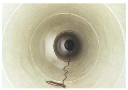
The picture on the left shows the distribution pipeline, after the coating was finished, getting more narrow from turbine to turbine. At the end of the distribution pipeline, the exhaust pipes for the acclimatisation were installed.
