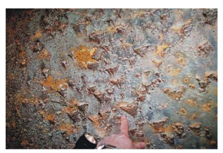
Large surfaces of the old coating, on a tar basis, were destructed by rust pustules. These pustules were several cm wide and high. In the bottom area, almost no smooth areas without pitting corrosion or perforations remained to be found.
