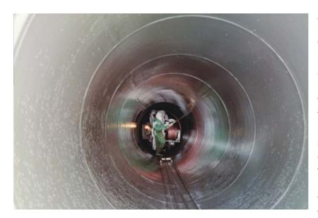
After the sandblasting had been checked, the working trolley loaded with Humidur® and the first layer of Humidur® was sprayed from the top to the bottom. The Airless spraying equipment was installed on the other end of the trolley, on which the two components of Humidur<sup>®</sup> were mixed too. Since the ambient temperature temporarily
