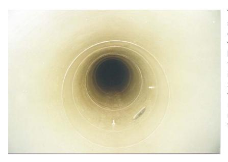
The picture on the left shows the finished coated pipeline after the trolley installation has been dis-assembled. On the right side there is an inspection manhole, (38 x 28 cm, oval), which was closed during the reparation works, by means of a wooden form.
