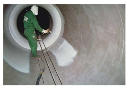
The first partial section in section 2 was a flat part of about 100 m up to the first bend (about 700 m²). The picture shows the application of the first Humidur® layer on the cleaned steel surface.
