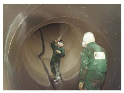
The two butterfly valves that flange the bottom side of the S-shaped armoured supply tunnel, and the diversion pipeline were disassembled. The picture shows the application of the second layer of Humidur® on the Sshaped supply water tunnel. The diameter is 2.4 m, the length up to the sliding room about 65 m. Since the slope was not steep here and not too long, it was not neces sary to use a trolley.
